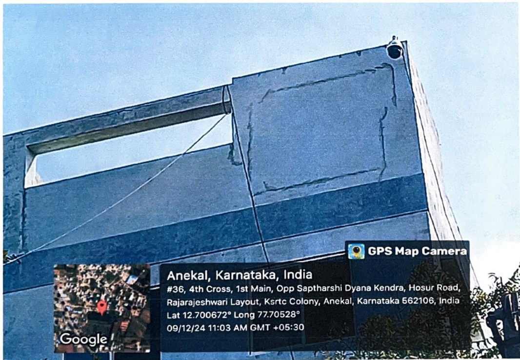
CCTV surveillance in entire campus
